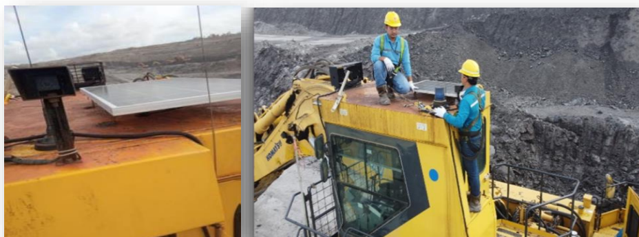
Solar Cell Installation
